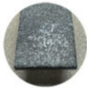
Figure 2: Clogged GritLock Surface
