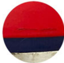
Figure 10: Cracking of Tri-Ply Seal
