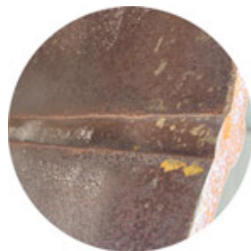
Figure 14: Weld Seam Along the Length of the Pipe
